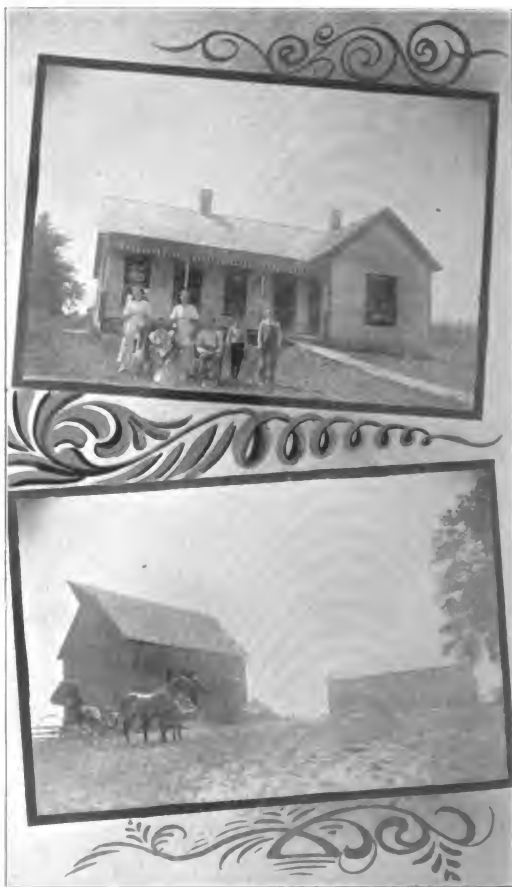
Residence, Family and Barns of Peter L. Miller, 5 miles southeast of Gibbs
